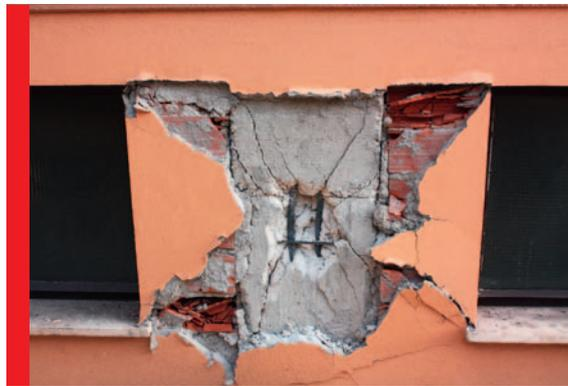
**Photo 11**Eclatement du béton, armature déformée, concerne peu de colonnes: *DD3*
